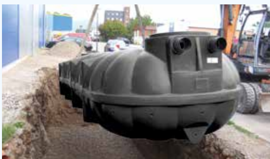
Installation NEO infiltrationstank 10 000 l
